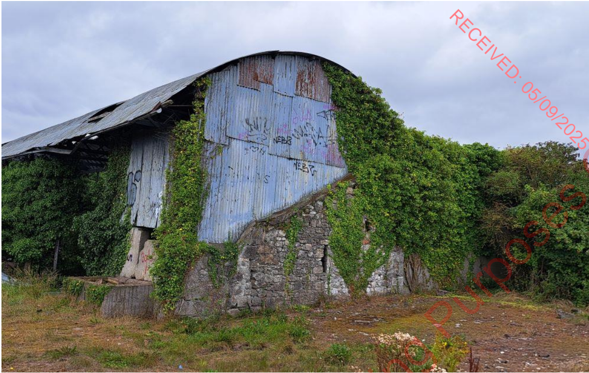
Plate 12.7 Remains of older farm buildings under modern developments
